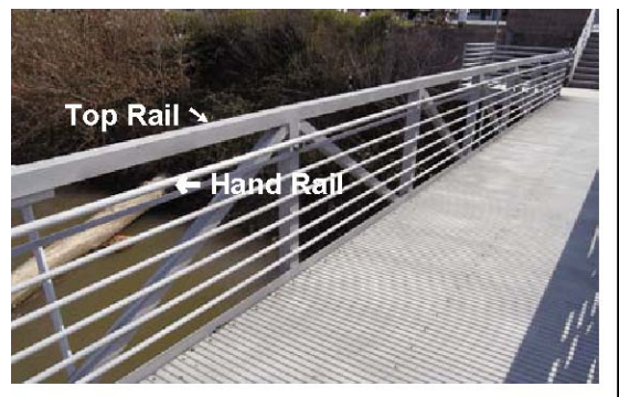
Guard Rail w/Hand Rail Meets 4" Sphere Test
