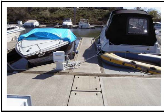
Non-Permanent Utility Lines Across Finger float
