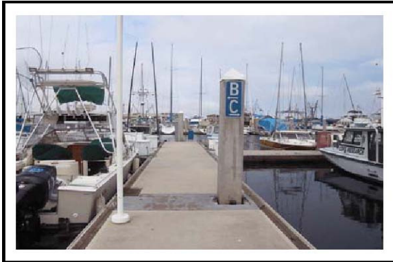
Pile Cap and Marker Signs
