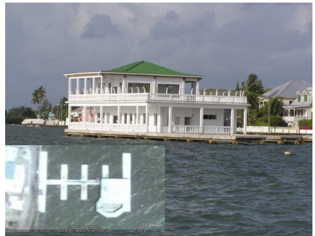
Bellevue overwater structure with docking facility
