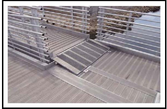
Toe Plate on Non-Accessible Gangway, or
